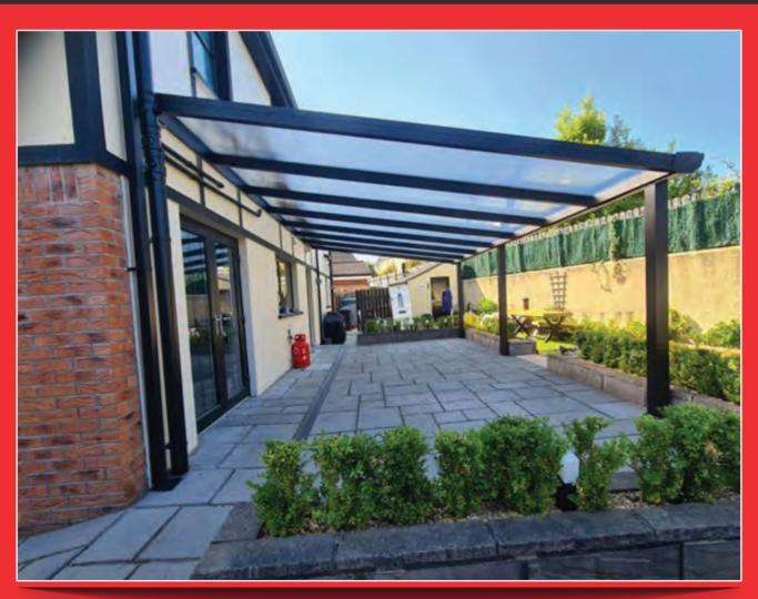
In their simplest form, our verandas are open sided (open on 3 sides), consisting of a roof abutted onto a house wall, and projecting up to 6m out from the building. A reinforced gutter at the lower veranda front is supported by a series of posts attached to the ground. Rain water from the veranda roof is fed into a downpipe, concealed within one of the support posts.
