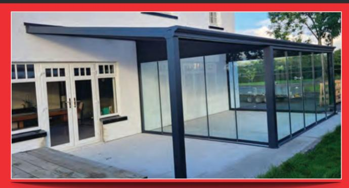
We can create a "Glass Room" on all or part of your veranda. In this example, a portion of the veranda reatains its open sides, while a section walled off with sliding glass panels creates a "Glass Room". Note that the "wedge" on top of the enclosed veranda sidewalls is solid
