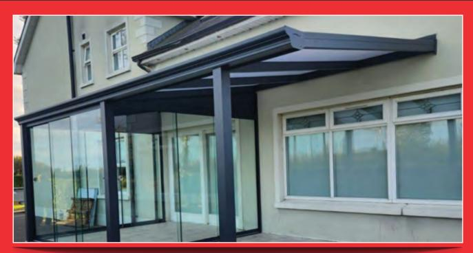
In most cases, the veranda front roof support posts are positioned at both front corners. The total number of front support posts fitted will depend upon the length of the veranda. In this case, one of the front corner support posts is
