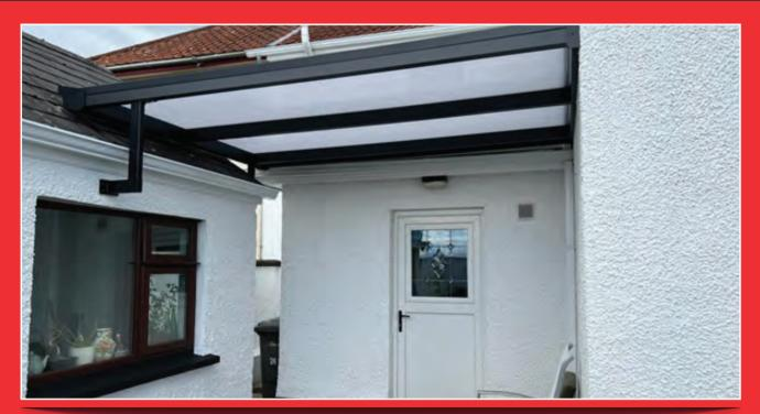
In most cases, our verandas are fitted onto your building, where the veranda backplate abutts onto your house wall and the lower front end of the veranda (where the veranda gutter is) is supported by vertical posts attached to the ground. In some cases, where this is not possible, the veranda roof is instead supported by custom made suitable wall brackets.
